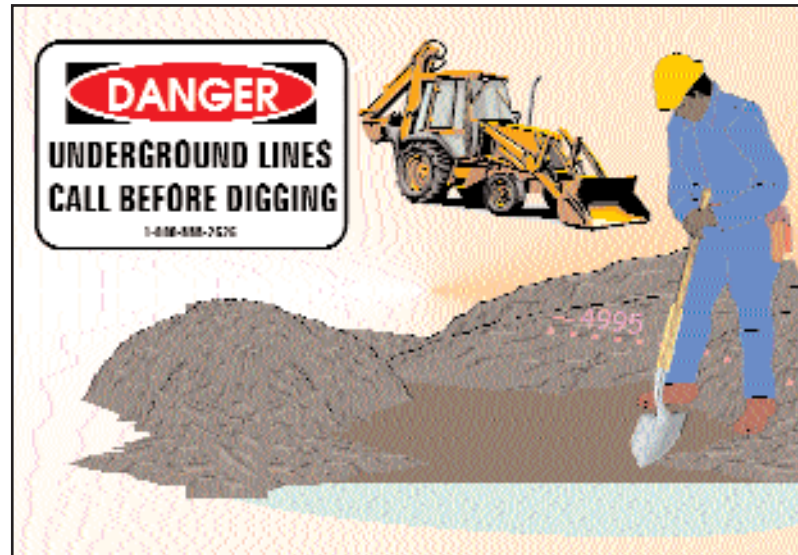
Fig. EH-4. Contact with buried utilities is just as hazardous as contact with overhead lines. It can cause explosion, fire, electrocution.
