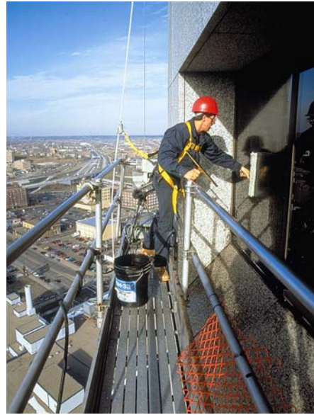
Lifelines must be designed to support 5,000 pounds per worker attached and protected against being cut or abraded (picture courtesy DBI/Sala).
