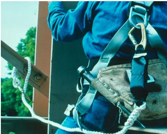
Unless approved by the manufacturer, snaphooks must not be tied back onto its own lanyard.
