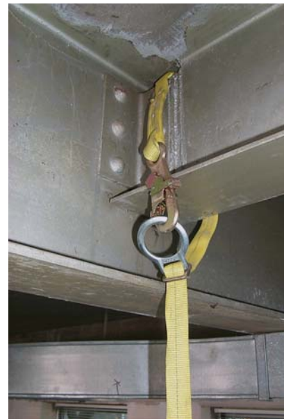
An example of an approved method to tie back a snaphook onto its own lanyard.
