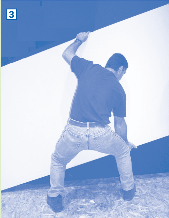
Figure 2. Proper horizontal installation sequence: (1) Raise edge of sheet, (2) grip with both hands, (3) hold in place with one hand and shift grip to bottom, (4) shift both hands to bottom, and (5) lift into position.
