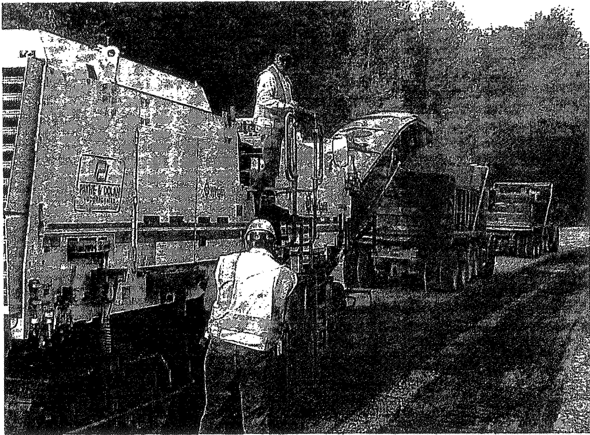
Figure 6: Operator and foreman, Foreman is operating right rear controls.
