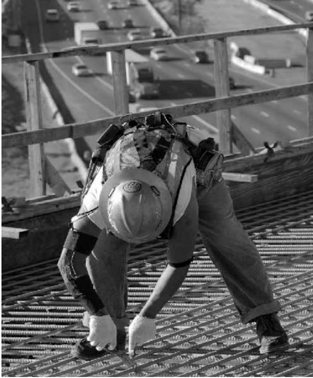
Figure 1. Rebar tying using pliers. Note the bent posture and awkward hand position.
