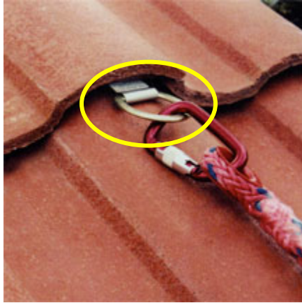
Figures 11 & 12 - Permanent anchors on completed roofs.
