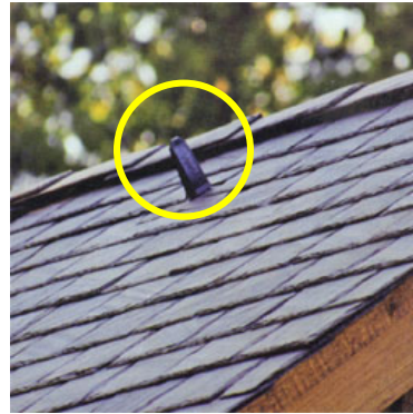
Figures 11 & 12 - Permanent anchors on completed roofs.
